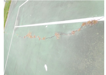
Northway Park and the Village tennis courts and the pickleball courts have cracks w/ weeds and worn surfaces that interfere with play.
